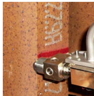
Chimney stone line-marking for correct installation
